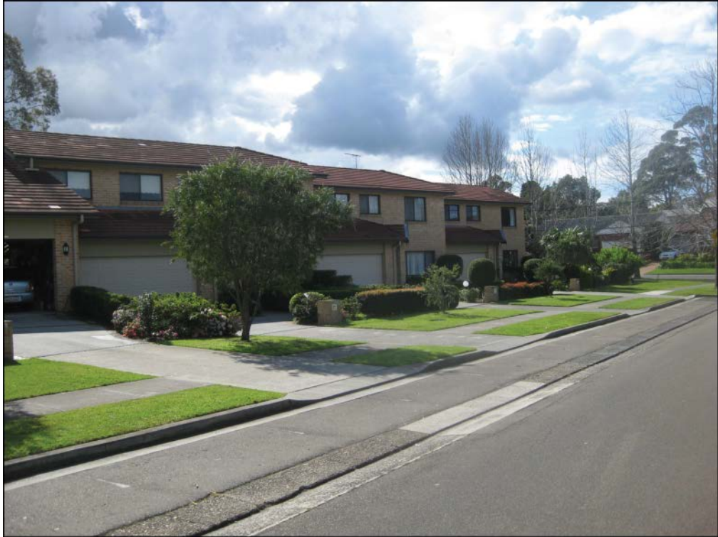
Figure 8: View east of townhouse complex.
